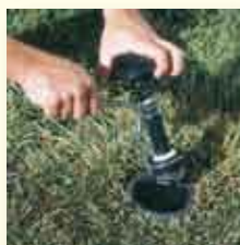
1. Remove internal assembly of existing sprinkler.
