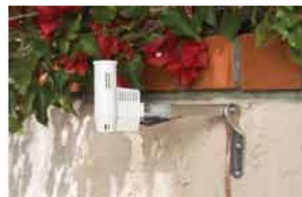
Rain/Freeze-Clik controls system operation during freezing temperatures.
