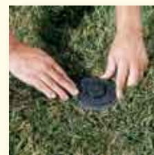
4. Install cap portion of ATR.
